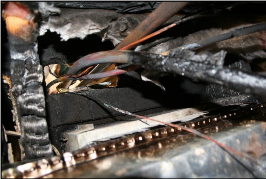
Figure 1 - View Looking Up at Sub Floor below Furnace
